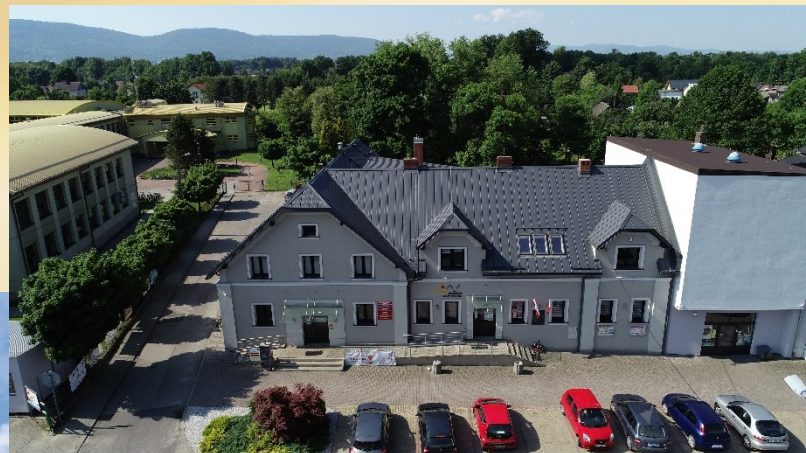
Fasada i parking
